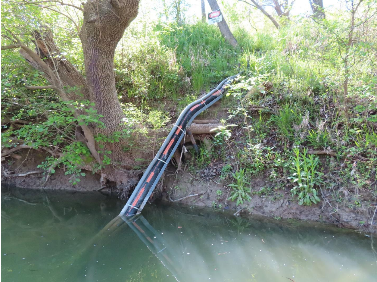
Figure 5. Location of an intake pump to supply water to an artificial 2 acre recreational lake at Mirasol Lodge LLC from the Pedernales River within the range of the Pedernales River springs salamander. Maintaining Pedernales River baseflows may be important in maintaining spring baseflows where the Pedernales River springs salamander is found.
