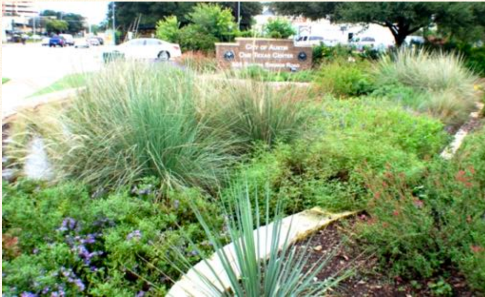
Bioretention pond outside Austin Watershed Protection building. Source: City of Austin website
